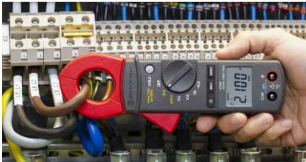
Fig 9- Rechecking faulty circuits
